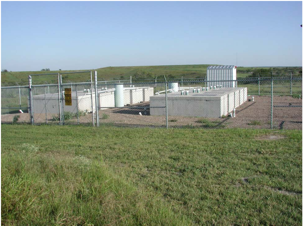
The Treatment Center Filter Beds at the Northbound Rest Stop
